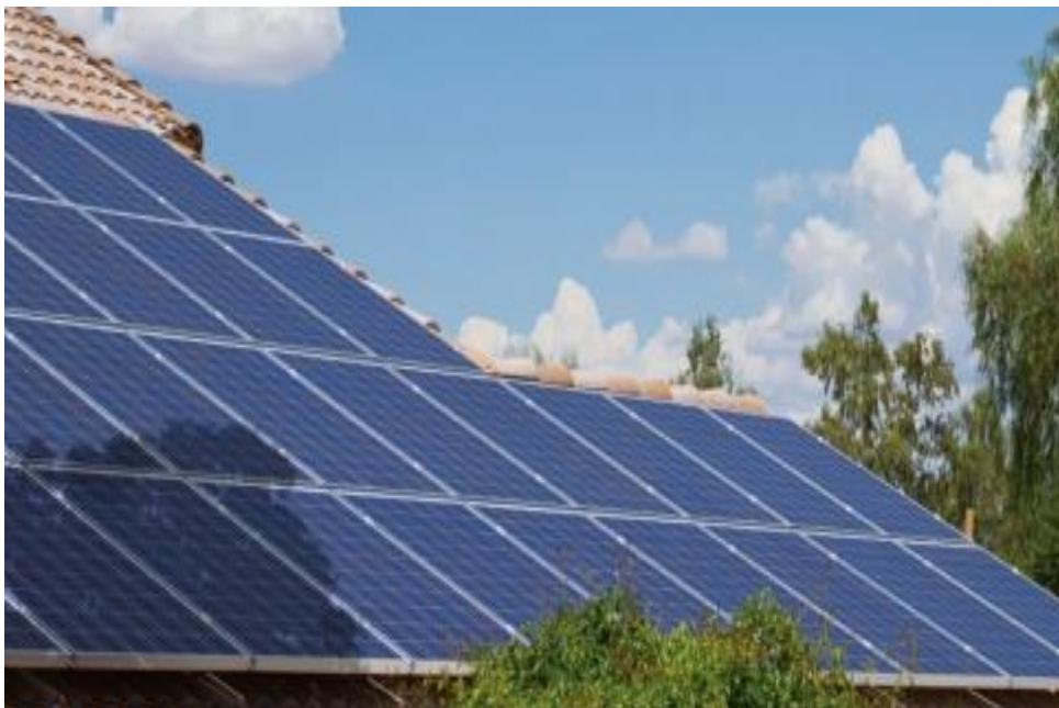
Fig. 1: Partial shading of PV module
