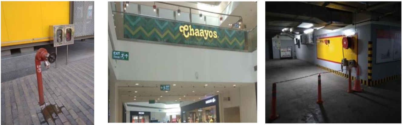
Figure 4.1.6 Fire exits in DLF Mall Of India
