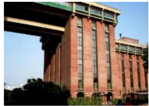
Fig.5.4 Brick cladding and ribbon windows
