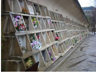
Figure 136-Concrete and marble columbrium rubble
