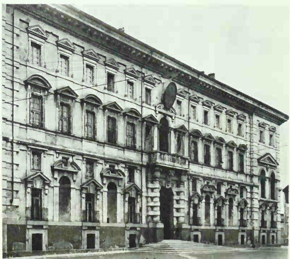
325. PELLEGRINO TIBALDI. Façade, Collegio Borromeo, Pavia. 1564. 83'6" × 236'
