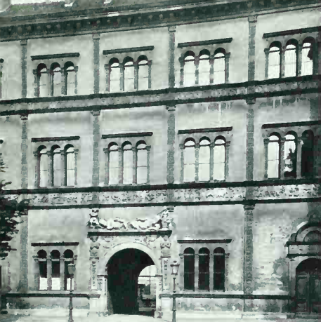
499. GABRIEL VON AKEN and ERHARD ALTDORFER. Courtyard façade, Wismar Castle. 1553. Height 57'
