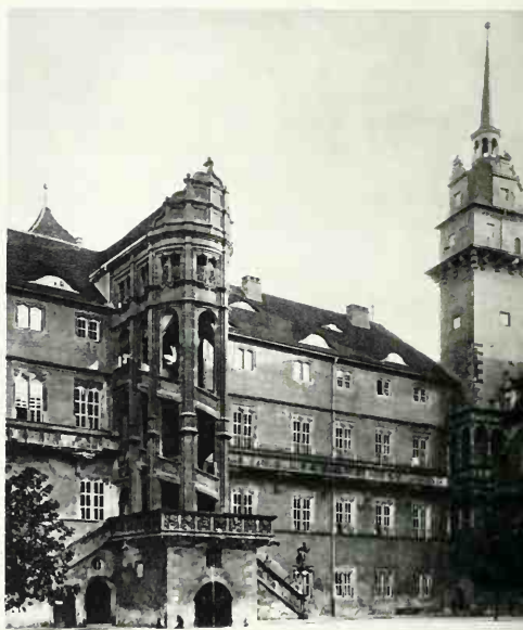
476. CONRAD KREBS. East wall, Courtyard, Schloss Hartenfels, Torgau. 1532. Length 179', height of projecting bay 89', width at ground level 26'4"
