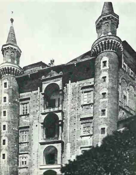
159. LUCIANO LAURANA. Loggia on exterior, Ducal Palace, Urbino. Total height of porches 50', width 13'
