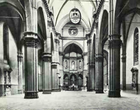
75. Interior, Cathedral, Florence. Begun 1296 (vaulting begun 1357). Height 145', width 135'
