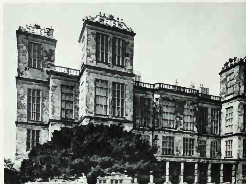
502. ROBERT SMYTHSON. Façade, Hardwick Hall, Derbyshire. 1590. Width 202'
