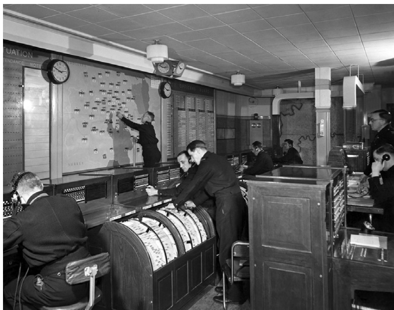
Figure 6.8 London Fire Brigade Headquarters control room, 1939.
