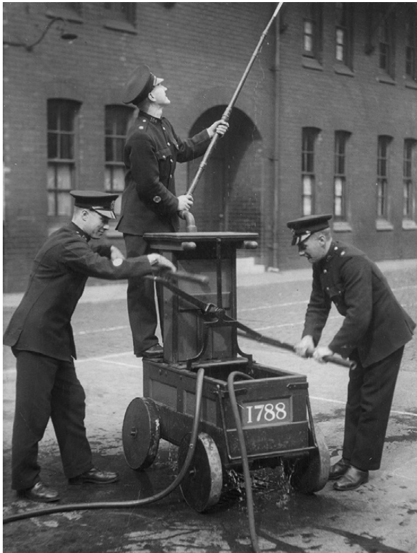
Figure 6.5 Hose pump operated by members of the Sunderland Fire Brigade in the 1930s. © Mary Evans Picture Library.
