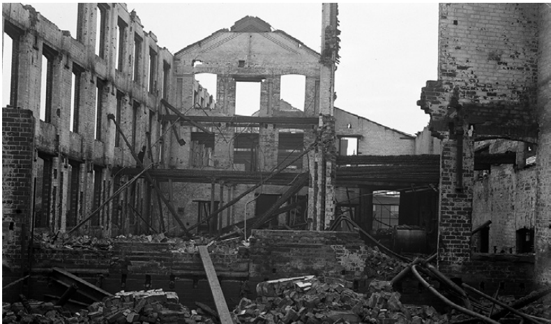
Figure 6.4 Massive fire damage at Battersby hat factory in Offerton, Stockport, after a fire in 1906, showing the extent of destruction, yet manufacture was stopped for only six weeks. © Mary Evans Picture Library.
