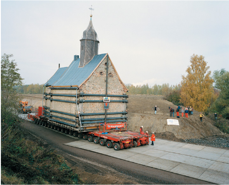
Figure 4.1 The relocation of the 800-year-old Emmaus church from Heuersdorf in Germany to the nearby village of Borna in 2007. The residents of Heuersdorf, a town that had to be abandoned to allow for the expansion of a nearby coal mine, protested for the safe relocation of their church to a new site. This relocation was a 12-kilometre journey that lasted for nine days. © Susanne Ludwig.
