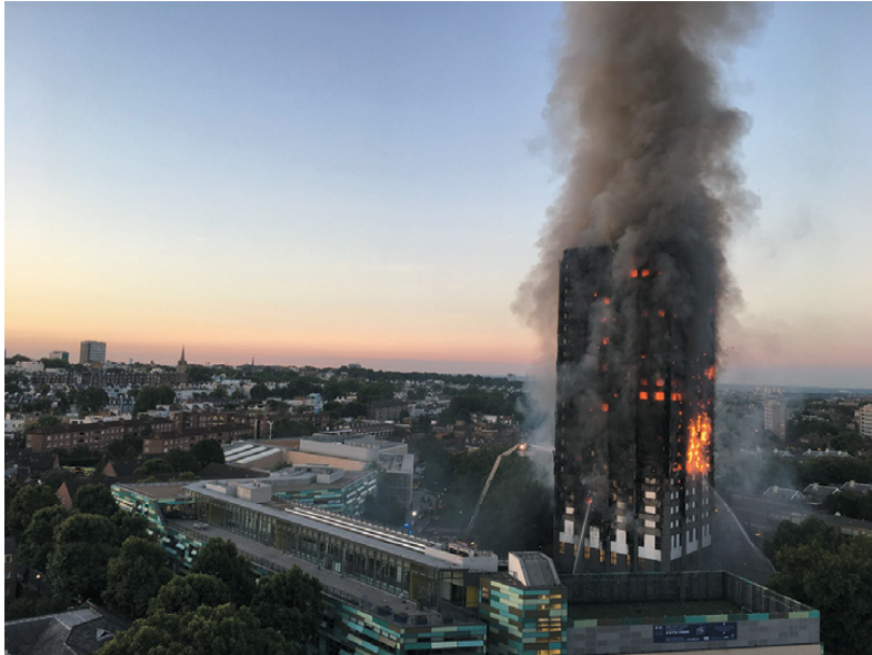
Figure 6.13 Grenfell Tower in flames, 14 June 2017. © Natalie Oxford/CC BY 4.0.
