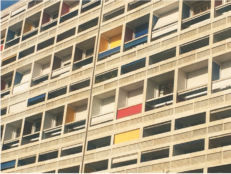
Figure 5.10 Le Corbusier's brise-soleil system at the Unité d'Habitation in Marseille, built 1947–52. © Marie Dumas.
