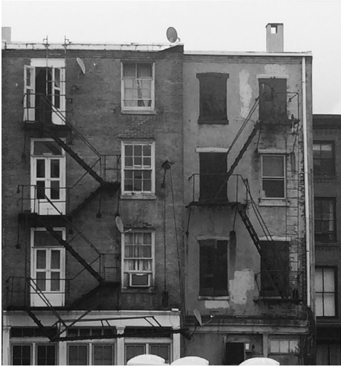
Figure 6.12 Steel fire escapes in Old City, Philadelphia. © Astero Klampatsa.
