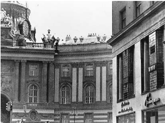
Adolf Loos, house on the Michaelerplatz, view of a detail of the Loos house together with the Hofburg at the other side of the Michaelerplatz.
