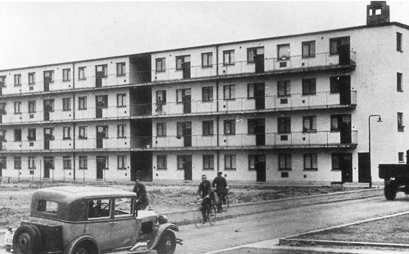
Blocks in Westhausen designed by Ferdinand Kramer. View of the north facade.
