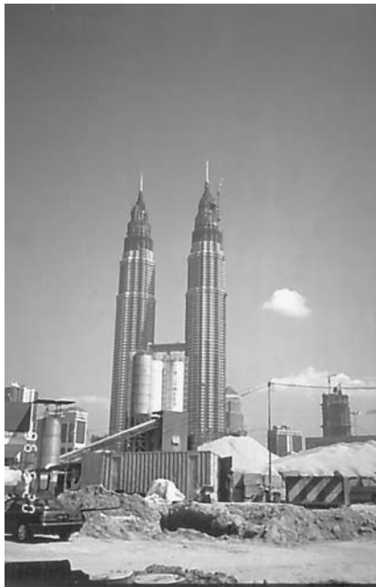
FIGURE 42.5 Towers with batch plant, Malaysia.
