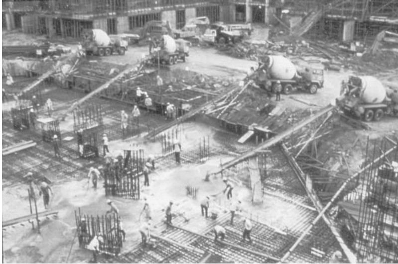
FIGURE 42.3 Concrete placing at Raffles City, Singapore.
