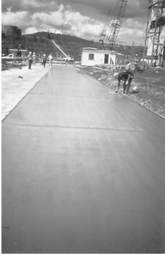
FIGURE 43.25 First pour of 32 MPa HVFA concrete in an apron slab at Mount Piper Power Station in New South Wales in 1991.
