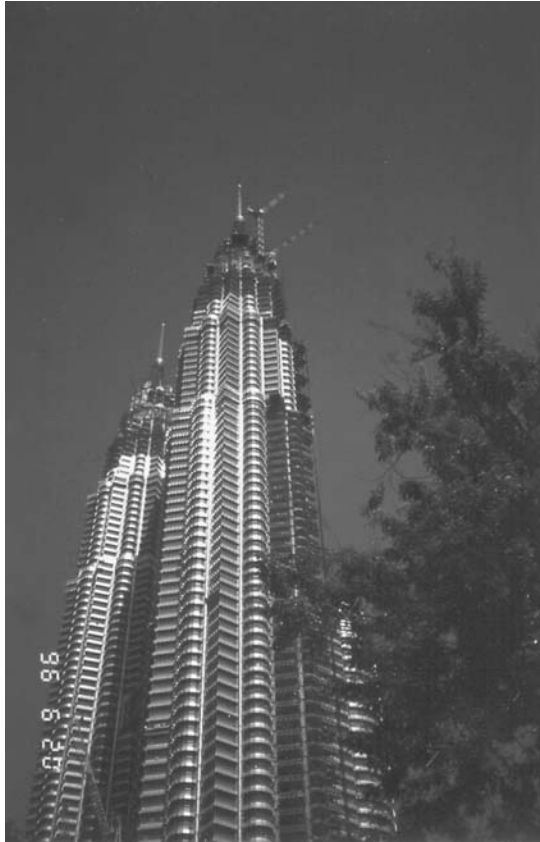
FIGURE 42.1 Petronas Towers, Malaysia.
