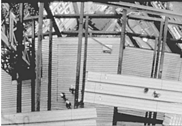
FIGURE 51.2 Composite steel–concrete floors, Grosvenor Place, Sydney.
