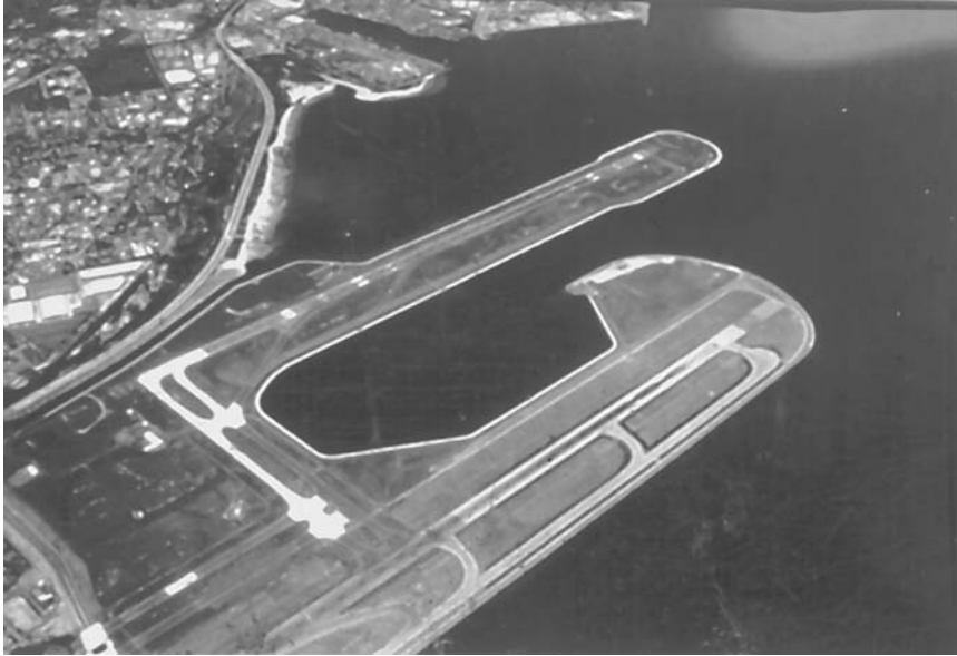
FIGURE 42.7 Aerial picture of seawall around Sydney Parallel Runway, Australia.
