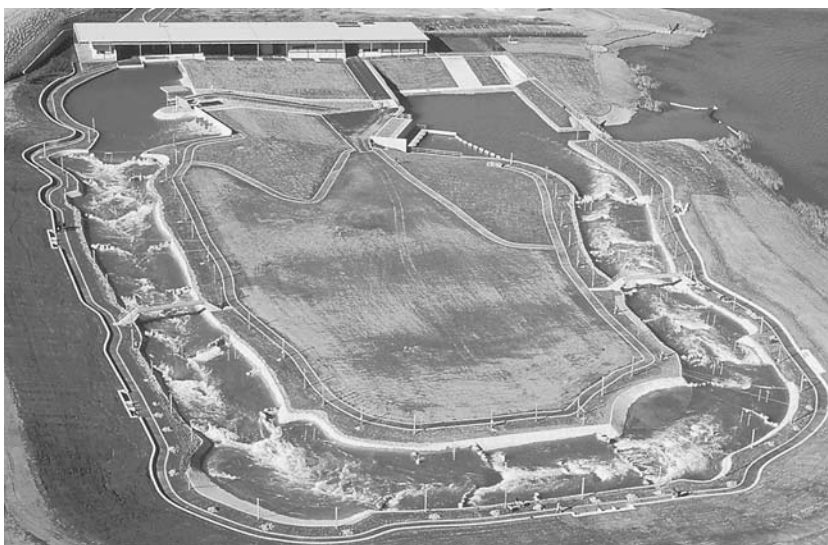
FIGURE 42.28 Aerial view of the Penrith Whitewater Stadium showing the complexity of forms, which favors the use of shotcrete (picture courtesy of the Sydney Olympic Co-ordination Authority).
