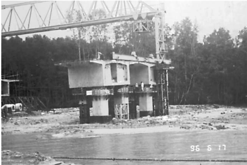
FIGURE 42.27 Construction activities at the Malaysia Singapore Second Crossway in 1996.
