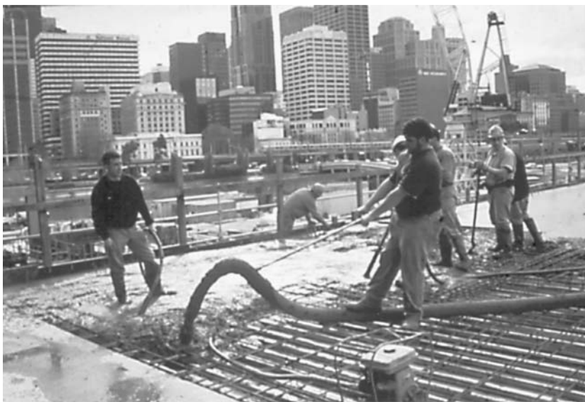
FIGURE 45.26 Crown Casino under construction in Melbourne Australia.
