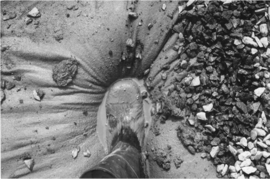
7.1 Non-woven geotextile over soft soil as a separator for crushed stones and a worker's boot.
