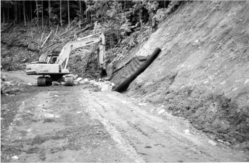
6.1 Cut-slope stabilization: geotextile filter and rock blanket.
