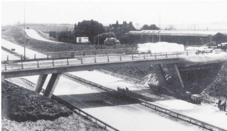
Fig. 6.9. Swanley bridge during plating operations.
