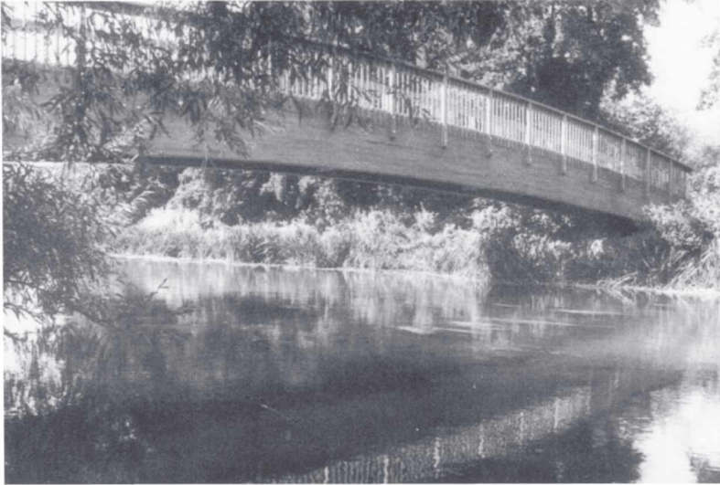
Fig. 7.12. Glulam hardwood footbridge.
