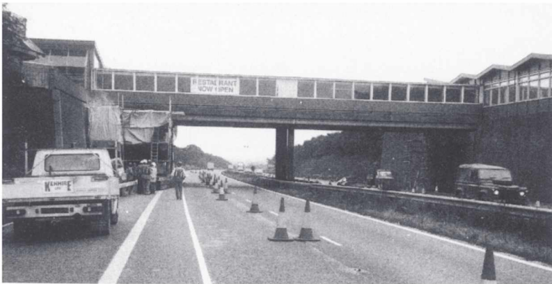
Fig. 6.8. Strengthening of a motorway structure whilst still in use.
