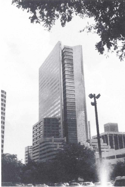
Fig. 1.5. Brickell Bay Office Tower, Miami, Florida; 28 floors, 4-sided structural silicone glazing.
