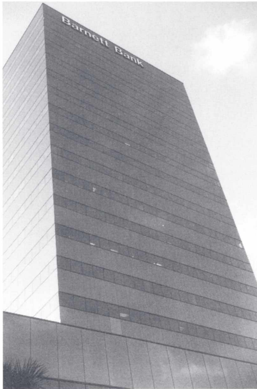
Fig. 1.4. Barnett Bank Centre, Miami, Florida; 15 floors, 4-sided structural silicone glazing.
