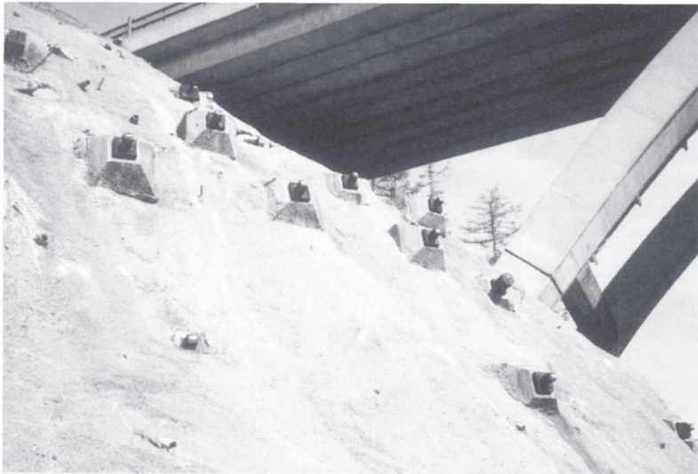
Fig. 7.6. Rock bolting in highway cutting.
