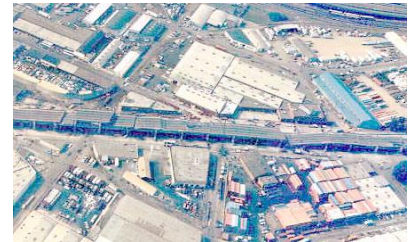
f / The collapsed section of the Nimitz Freeway.
