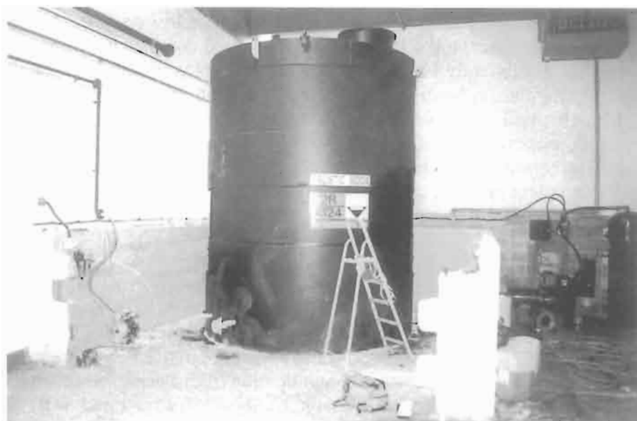
Fig. 2. Failed plastic tank, showing the bund wall in section (the front part was removed by the Fire Brigade). The jet of caustic soda flew from the tank wall near the right-hand edge in the figure, just above the top of the bund wall. It rose upward from a small crack in the weld, and landed some 4–5 m away from the exit point.
