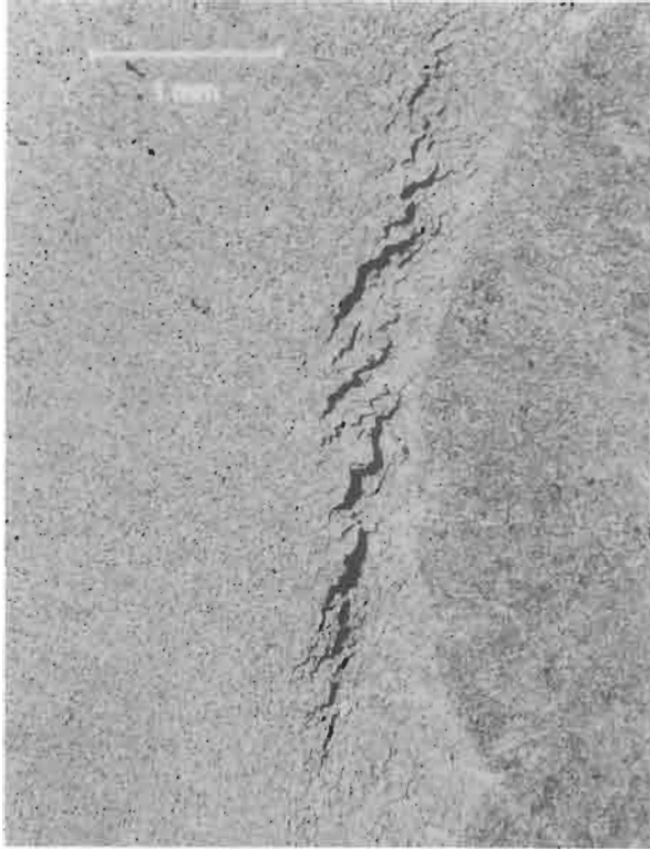
Fig. 7. One of the clusters of cracks in the HAZ on the reducer side of the weld joining the X-side reducer to the 8 in. pipe HAZ. The whole cluster is about 3.8 mm top to bottom.
